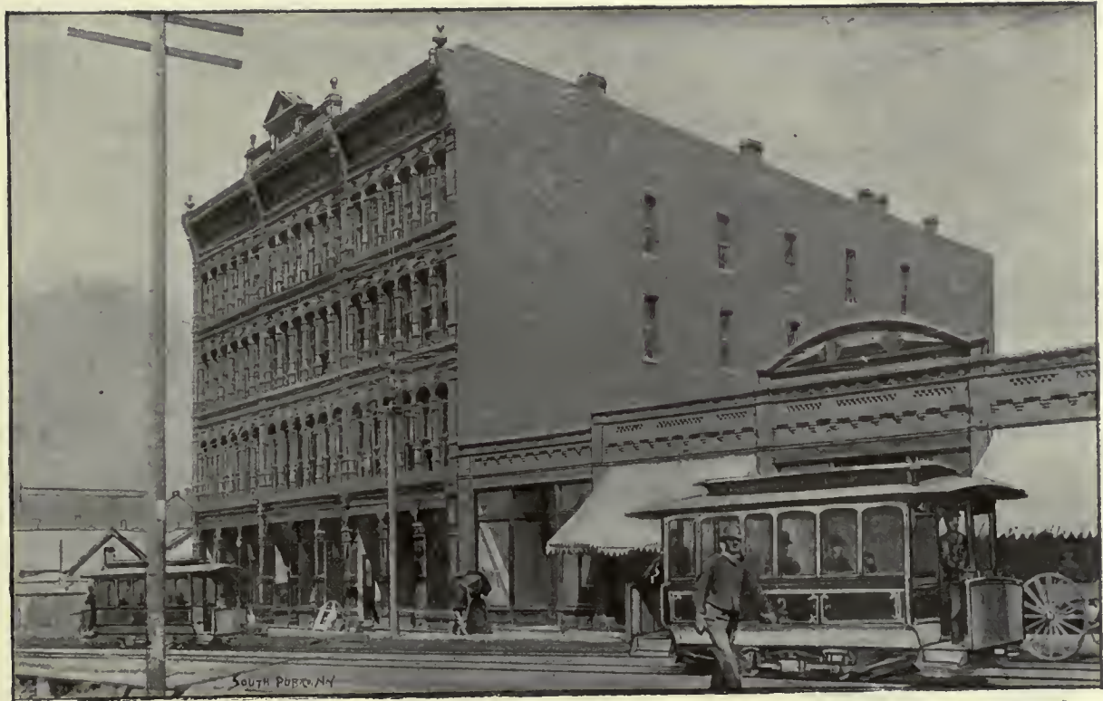
IRON FRONT BUILDING.
